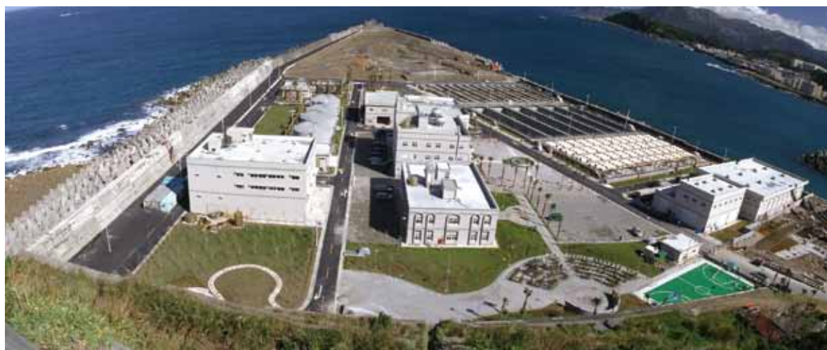
📍 The sewage treatment plant in Hopin Island, Keelung.
